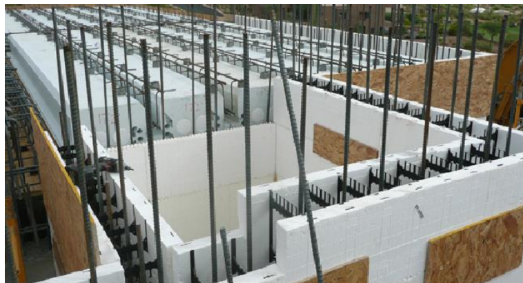
Figura 3.15 Cofraj termoizolant, sistem Amvic http://www.amvic.ro/img_pliant/a.jpg
